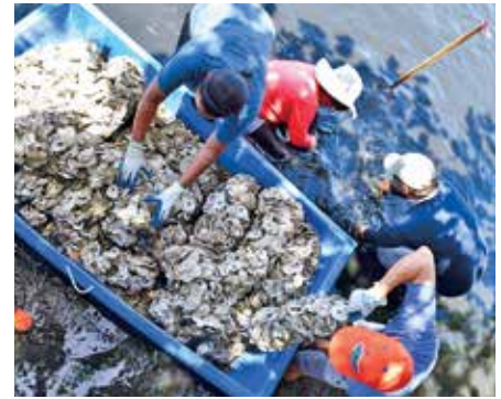
Volunteers turn bags of oyster shells into a structure engineered by Florida Tech to lure oyster larva and serve as a barrier to shore erosion.
