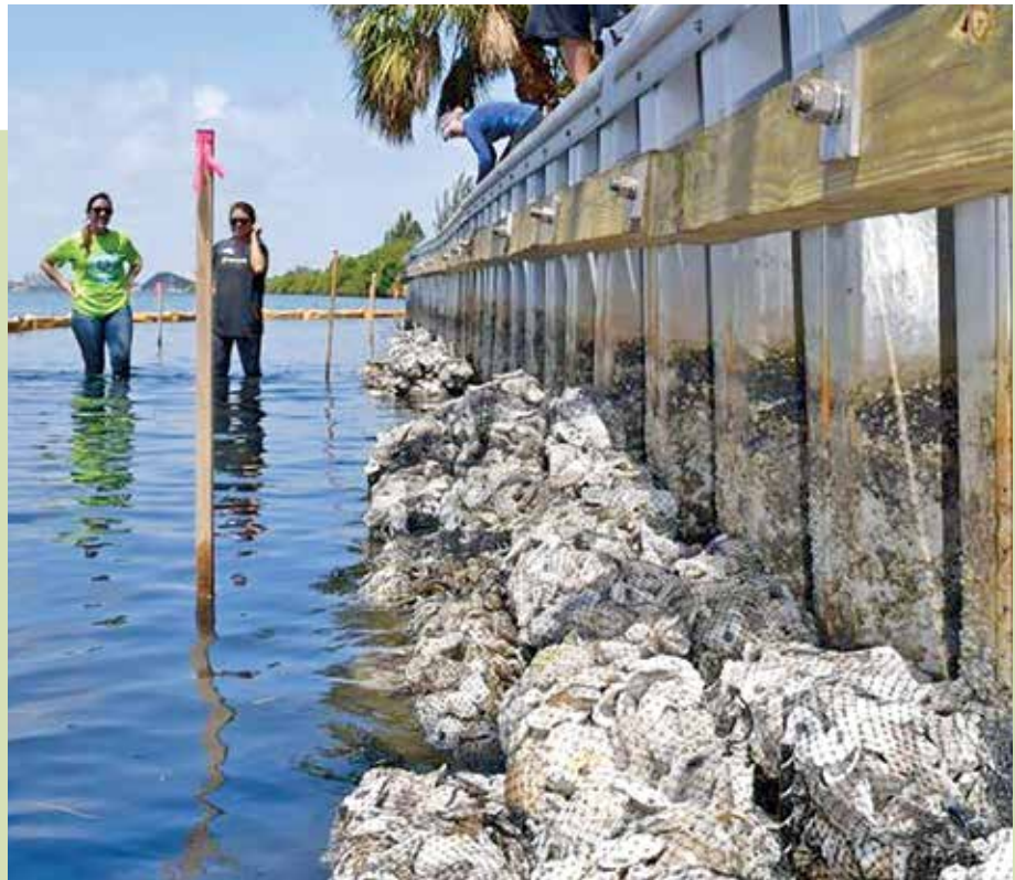
Volunteers turn bags of oyster shells into a structure engineered by Florida Tech to lure oyster larva and serve as a barrier to shore erosion.
