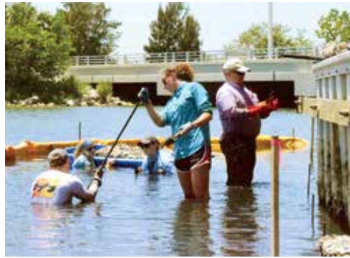
Volunteers turn bags of oyster shells into a structure engineered by Florida Tech to lure oyster larva and serve as a barrier to shore erosion.
