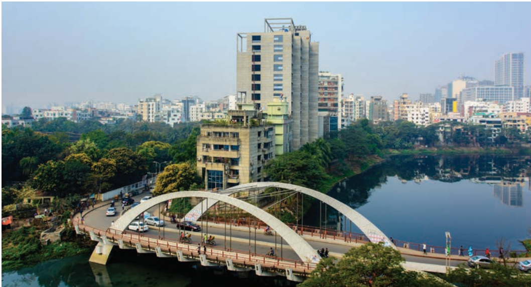
Bangladesh, one of the fastest-growing countries in South Asia, is expected to experience a rise in energy demand. This photo shows a recently constructed high-rise building in Dhaka, Bangladesh.
