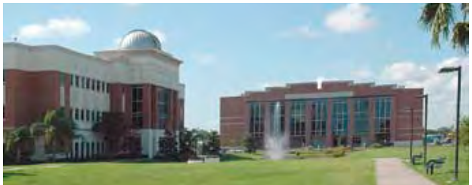
The new Harris Center for Science and Engineering, adjacent to the F.W. Olin Physical Sciences Center, is nearing completion.
