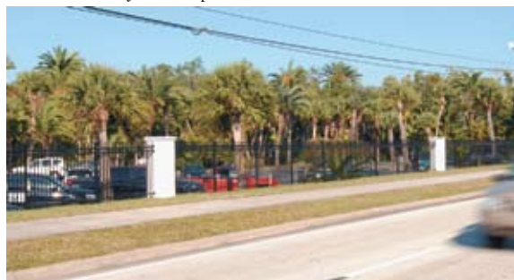
New Babcock Street fence delineates campus border.
