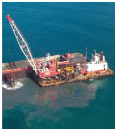
Feature: The extraordinary construction project at the Port of the Americas.
