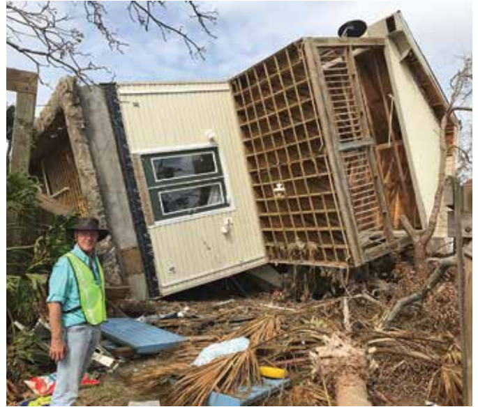
Jean-Paul Pinelli evaluating an overturned house in Mexico Beach, Florida, after Hurricane Michael
