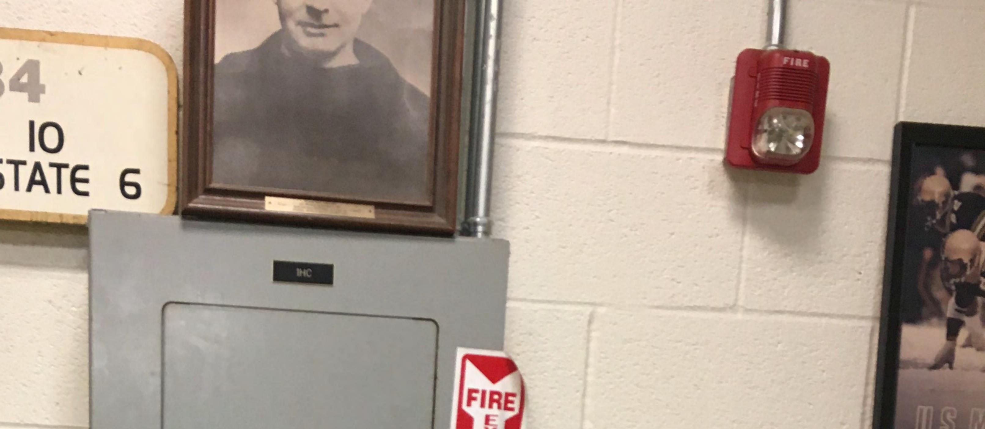
Electrical/fire hazard: blocked breaker panel and blocked fire extinguisher
