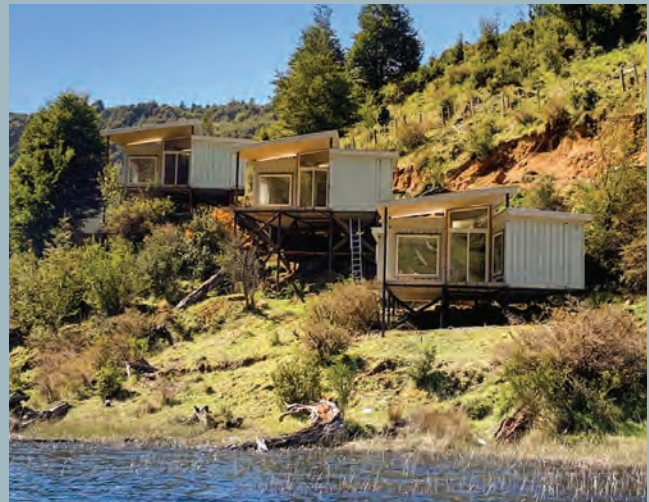
Construction on the Eko Patagonia resort
