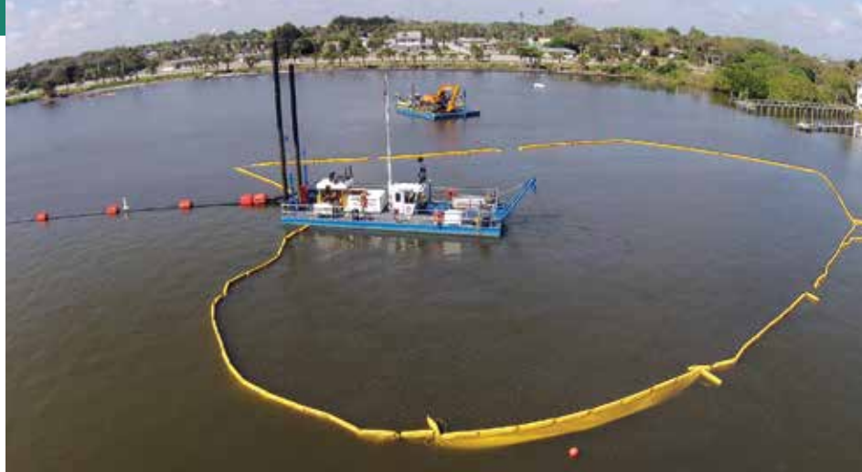
Dredging Turkey Creek. The platform holds a hydraulic pump that dips into the lagoon and essentially vacuums up the muck. It is siphoned through a pipeline to a spoil site on the riverbank where the offending muck particles can settle, and then the clean water left over can be pumped back in to the lagoon.
